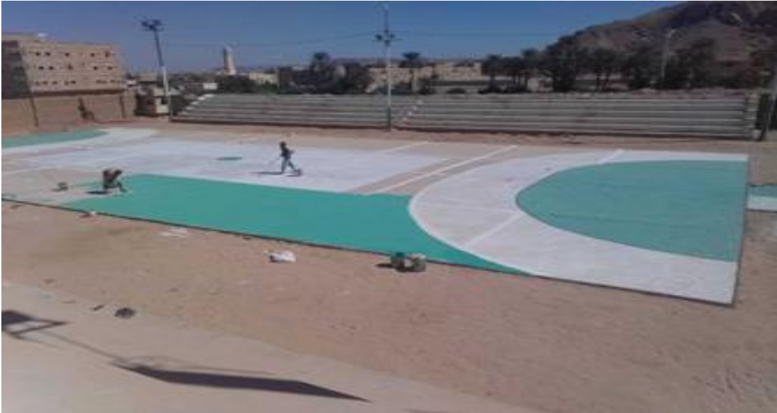
Painting and Marking Volleyball/Handball Ground
